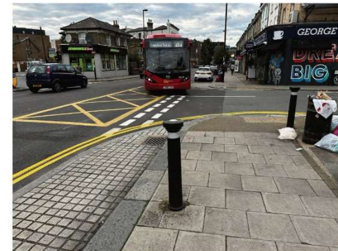
Paved overrun area The use of contrasting silver-grey granite setts and position of the road markings help to avoid the carriageway appearing excessively wide.
