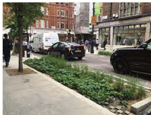
Repurpose 'baggy space' for greening and SuDS Hatched areas often present opportunities for planting, trees and SuDS.
